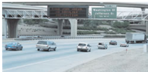
Variable message signs are a tool to help manage traffic.
